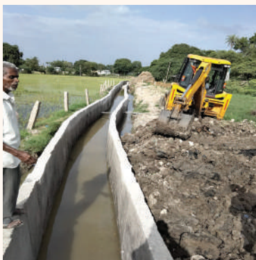
Construction of open drain
