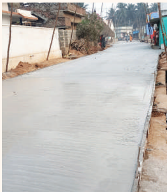
Rajayyapeta road work
