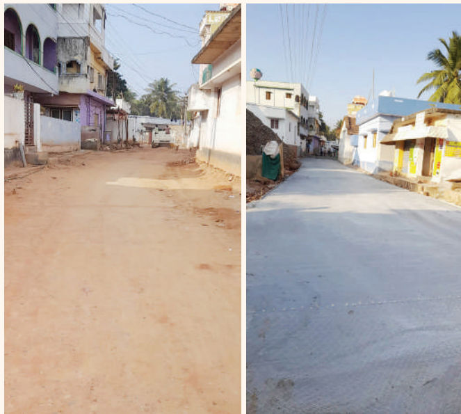
Peddateenarla CC roadwork before and after
