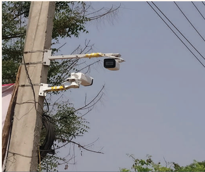
CC Camera installation for security
